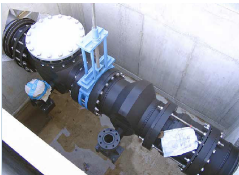
Fig 11: Example of a Sewerage rising main chamber with puddle flanges each end, knife gate isolation valve, Pressure drainage tees, dismantling joint and CCTV access point. All manufactured in PE except for the blank flange and the knife gate valve
