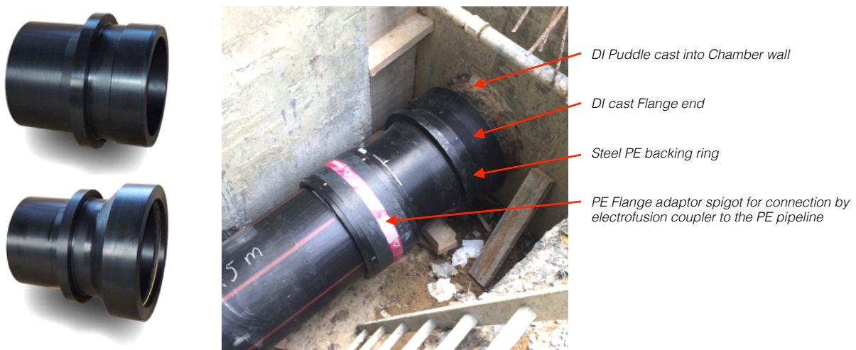
Fig 9: Example of a PE socket transition fitting. After connection to the PE pipe, the transition fitting is encased in concrete anchoring the transition fitting via the puddle flange to the DI pipe and the chamber wall
