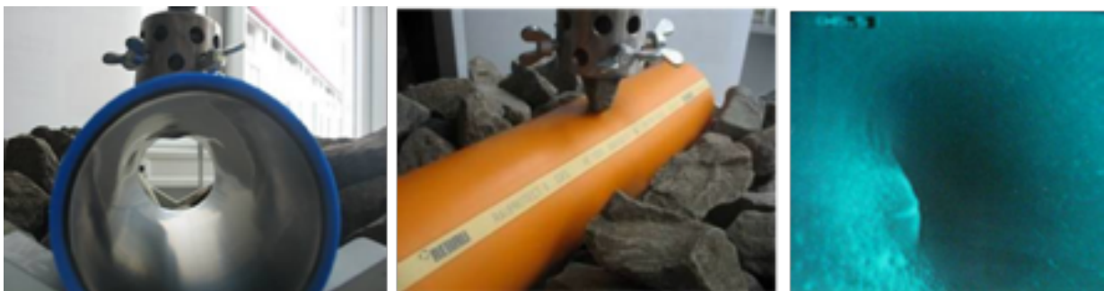
Figure 3 - Typical lab examples of point loads on PE pipes, and CCTV camera showing point load in service
